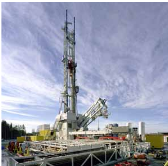
Dublett drilling, Kirchstockach, Germany
