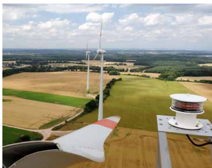
Wind farm Selmsdorf. Germany, obstruction lights
