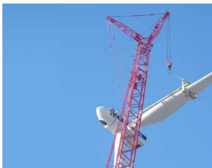
Wind farm Everswinkel in Germany, rotor blade assembly
