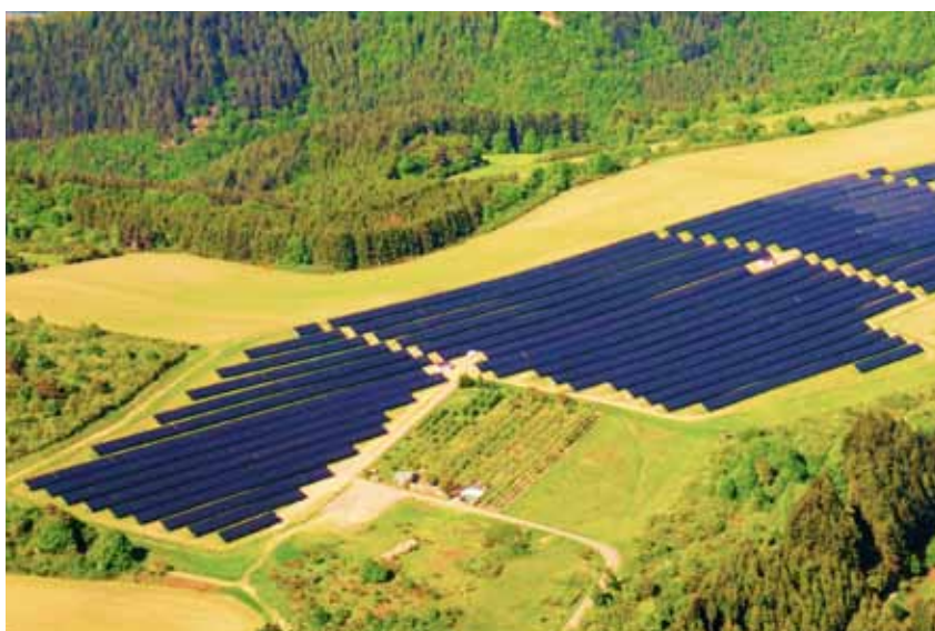
Photovoltaic plant Leiwien, Germany
